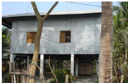
Photo 2.3.1 (c): New style of Govt. Sanctioned Rakhain House
