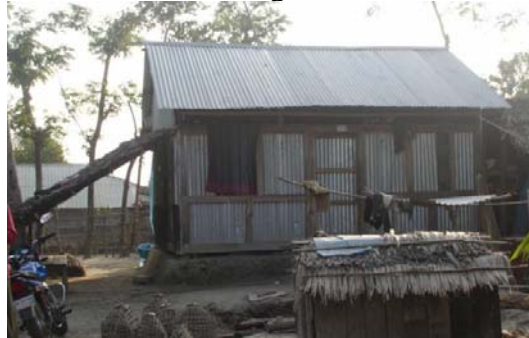
Photo 2.3.1(b): Rakhain House constructed like Bengali Houses
