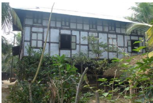
Photo 2.3.1 (a): A Three storied Rakhain House
