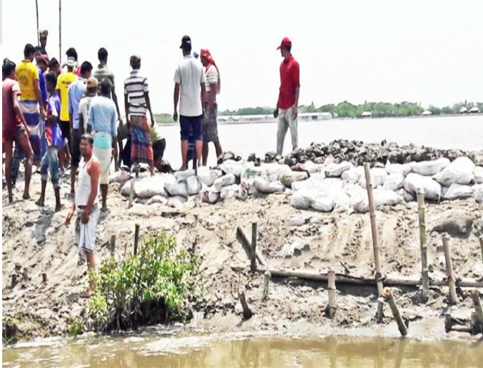
Photo: People repairing embankment
