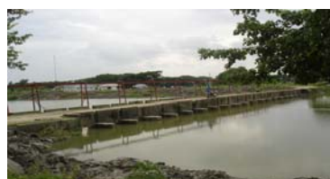
Bhabadaha Sluice Gate: Entrance point for people's pain
