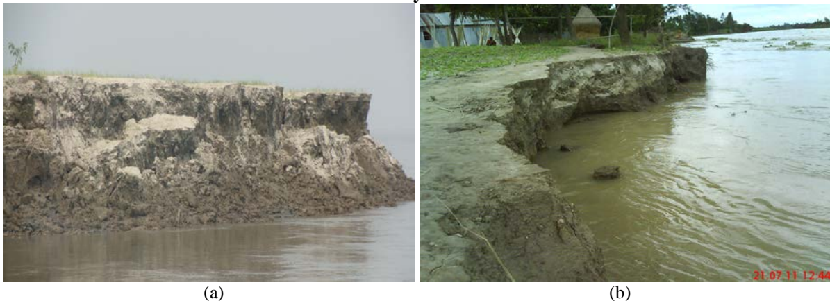
Photographs 1: (a) Mass wasting in a distant place from homestead and (b) erosion nearby study area
